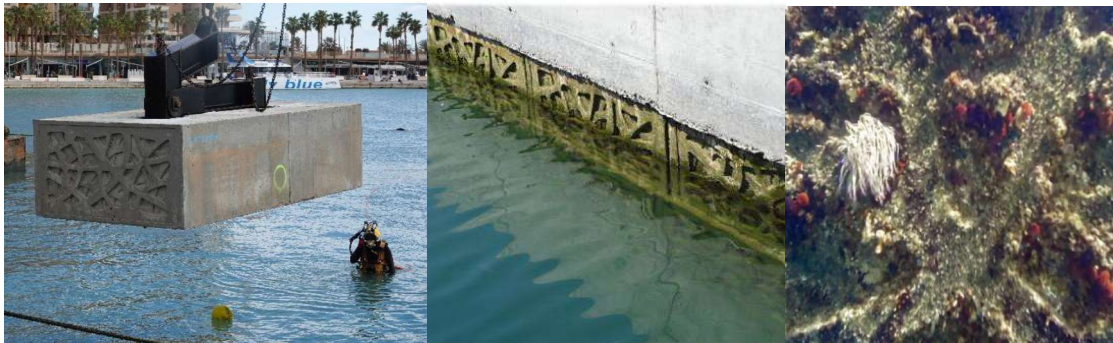
Figure 4. IGY marina vertical breakwater, designed with EONcrete Mass Concrete Blocks. Left – at installation; center – 3 months post-installation; right – 13 months post-installation.
