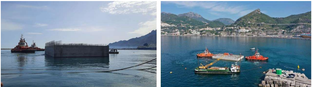
Figure 5. Concrete structure transportation from the construction site to its final position.
