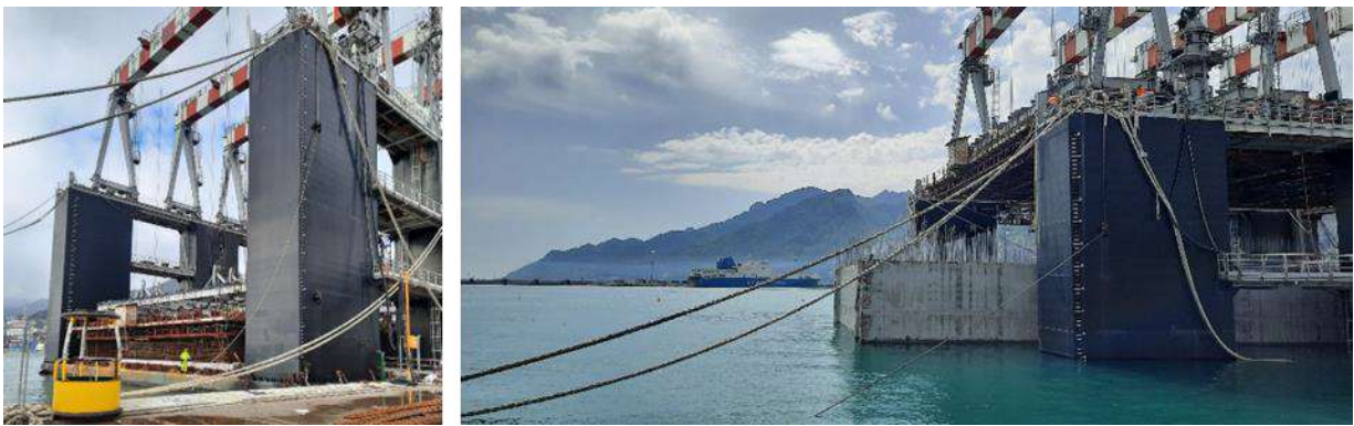
Figure 4. Construction of the concrete caisson up to +0.80m in the Dario dry dock.
