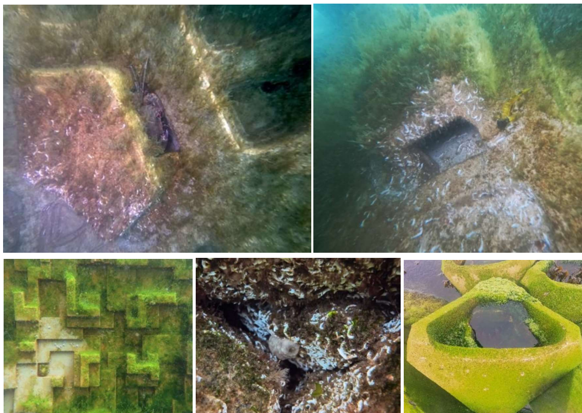
Figure 6. Biological development 3 MPD; (A) A crab of the specie Necora puber that found a shelter inside the Mangrove seawall pocket, the wall is covered with red algae (B) The dominant observed green algae ( Ulva sp. and Enterophormia sp.) covering an Azuri seawall pocket with Pomatoceros sp. polychaetas and a small Tripterygion delaisi fish. (C) Azuri seawall covered with the dominant green algae species, with Barnacles and a Limpet on the clear grazed area. (D) Pomatoceros sp. polychaetas and a Phallusia mammillata tunicate within the CL cavity. (E) CL unit in low tide covered with Ulva sp. algae.
